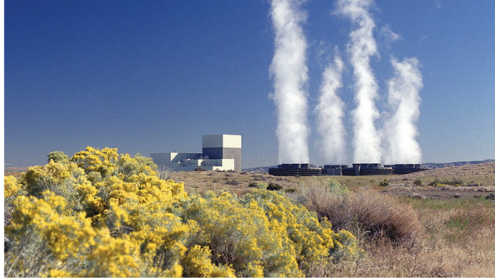
The Columbia Generating Station (Image: Energy Northwest)
